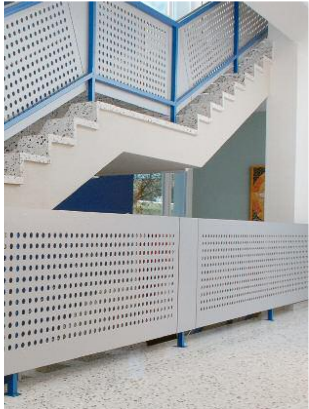
Staircase railing-enlarged holes in Max Alucompact42
