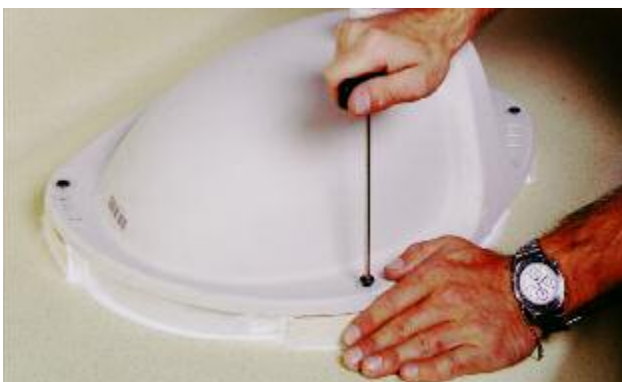
3. Glue the basin in with PUR glue and screw in as in the diagram.
