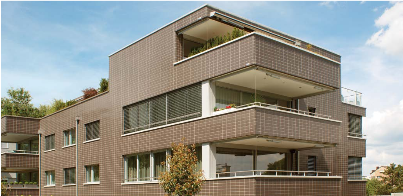
Apartment building, Kilchberg, Switzerland Architect: Horizon Architektur + Bau AG, Zurich, Switzerland Products: Chroma II, special colour
