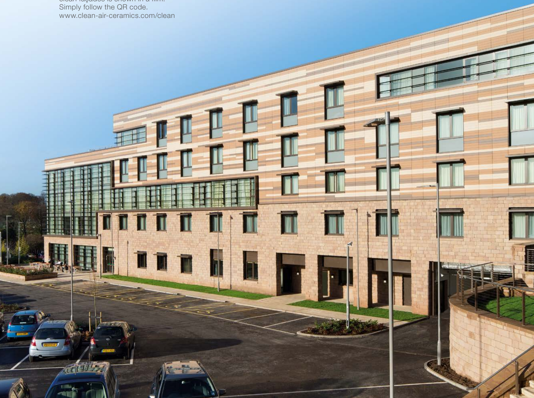
Orchard Hotel, Nottingham, Great Britain / Architect: RHWL Architects, London / Products: KeraTwin® (K20), special colours, clamp fastening
